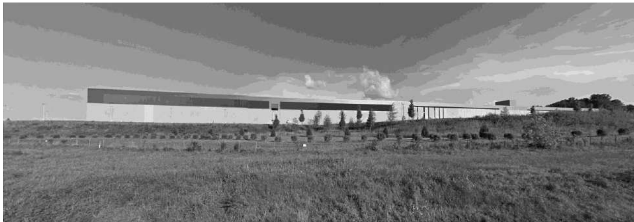
31.13.29.232 facebook data center, forest city , north carolina, us (photo: google streetview)
